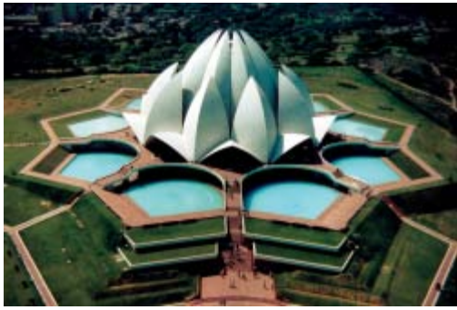
The Bahá'í House of Worship in New Delhi, India. 29 September 1989. © Bahá'í International Community. Bahá'í Media Bank
